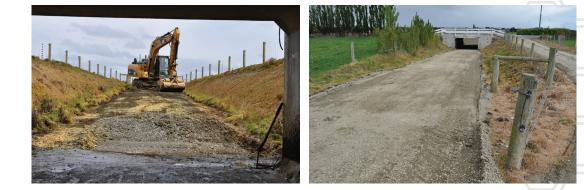
Remove overburden, apply GAP20 base aggregate and roll
